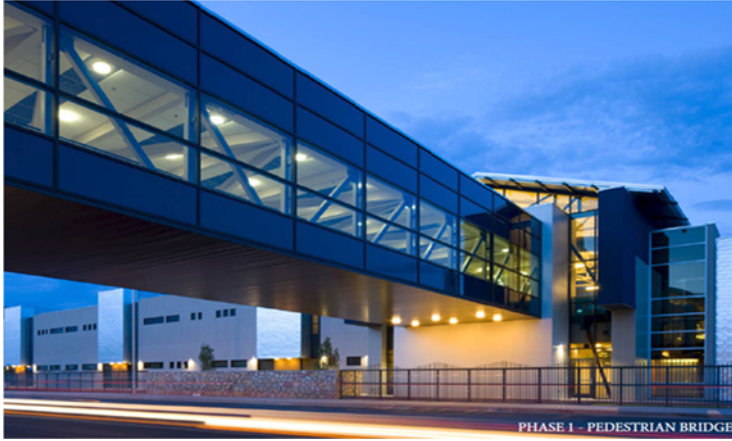
Las Cruces HS Administration and Pedestrian Bridge
