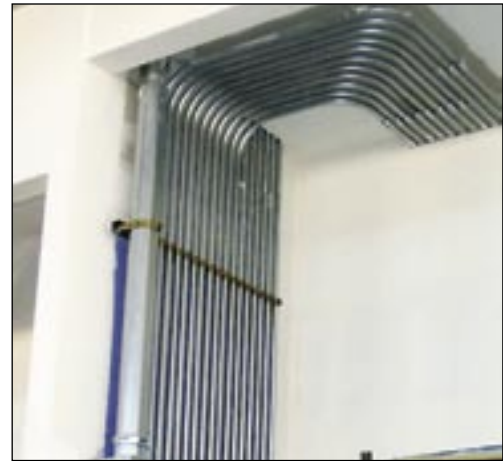
Bradley Harrison/Theco's award-winning electrical conduit work at Belen Career Academy.
