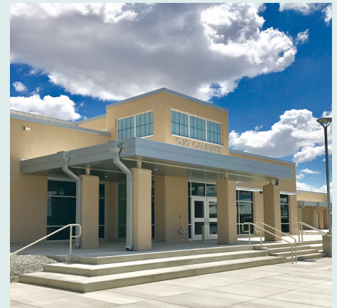
Ojo Caliente Elementary School(P14-018), © 2017 NMPSFA, All rights reserved.
