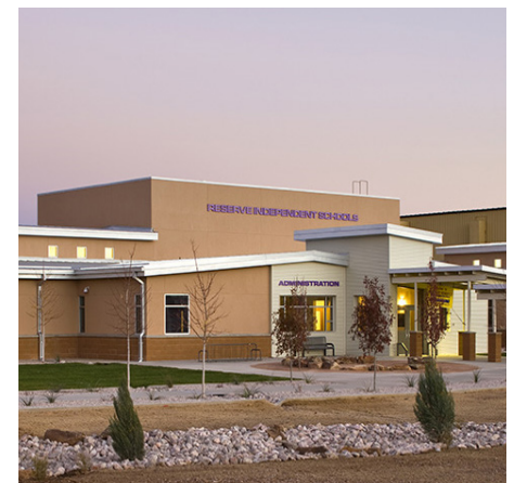
Reserve Combined School(P14-022), © 2016 Greer Stafford/SJCF Architecture, Inc., All rights reserve. Photo by Patrick Coulie Photography.
