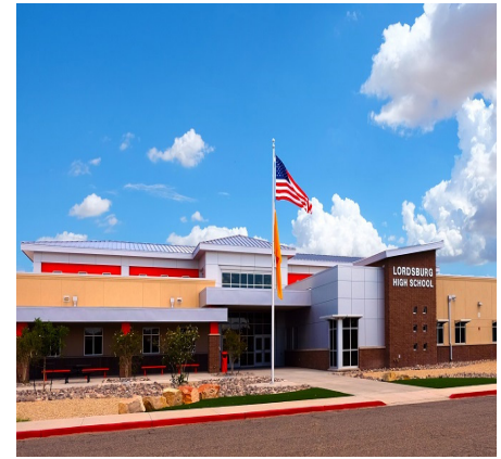
Lordsburg High School(P14-017), © 2017 HB Construction, All rights reserved.
