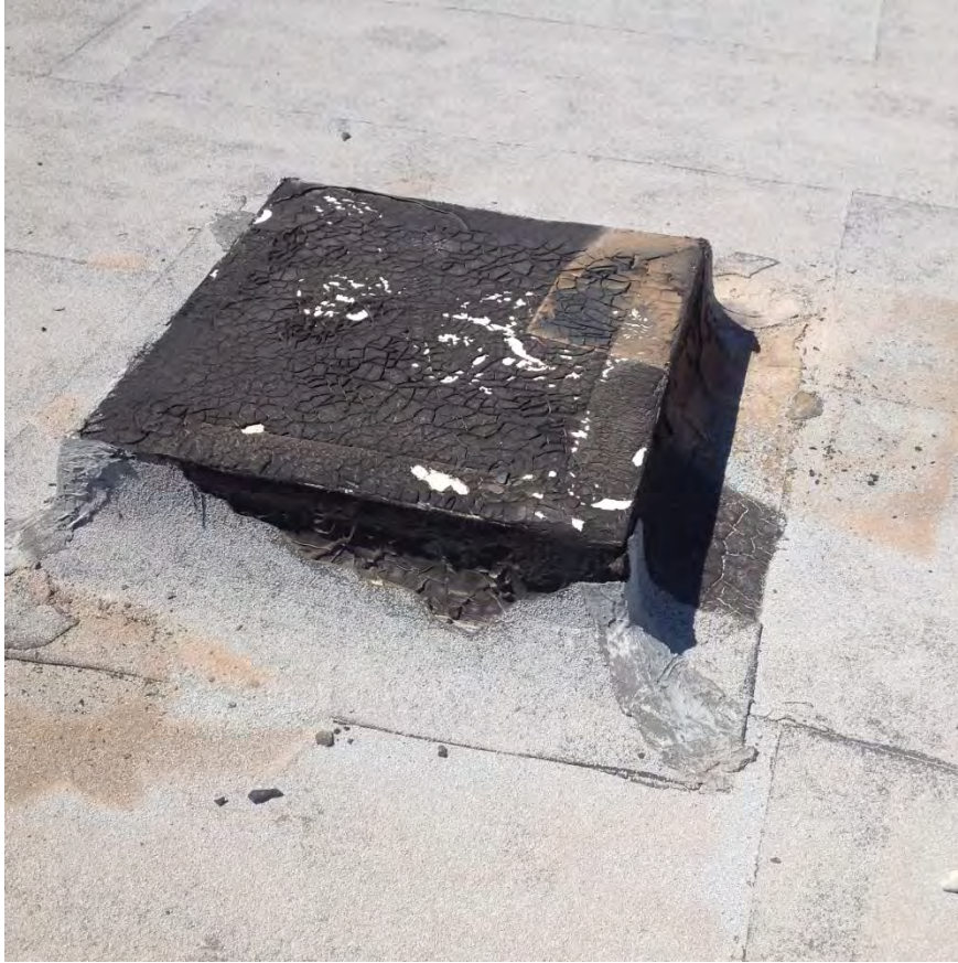
Existing abandoned curb(s) from previous evaporative units
