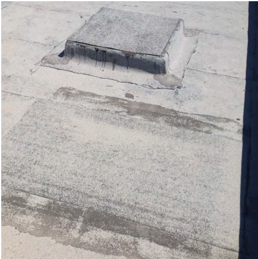
Existing abandoned curb(s) from previous evaporative units
