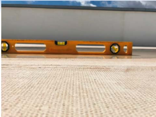
Photo No. 28 – Depicts one of numerous measurements taken by NMRC indicating there is no slope to promote positive drainage for this roof system. This generally does not meet industry standards and benchmarks for best practice, does not meet minimum code requirements for the year the building was constructed, and does not meet warranty requirements for this or any modern roof system manufacturer.
