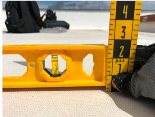
Photo No. 29 – Depicts one of several locations where slope was measured to be less than 1/8-inch per foot, likely at portions of the roof that may have added crickets to direct water away from corners.
