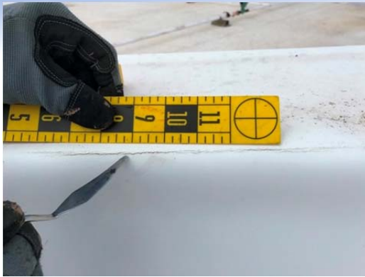
Photo No. 22 – Depicts detail view at a split in the membrane wall flashing, likely a result of fatigue by cyclical movement induced by wind and/or building movement, as well as exposure at the parapet transition.
