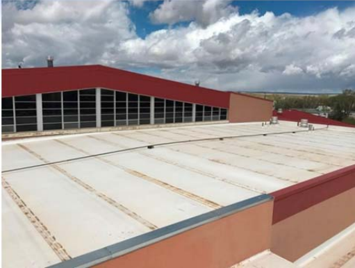
Photo No. 37 – Depicts overview at Roof Area 3 that is a Firestone brand TPO membrane, which is very different than the other field areas of the roof. This roof was found to be generally in good condition and has adequate slope for drainage.
