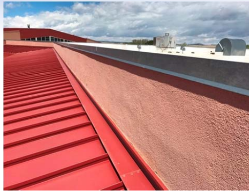
Photo No. 14 – Depicts a large portion deconsolidated and delaminated stucco wall cladding adjacent to a sheet metal roof system. This location appears to have been installed with a proper weep screed; however, the stucco does not appear to be well adhered, and may be delaminating from the assembly. Moisture that is trapped within this system may enter the wall and behind the roof at unsealed joints within the WRB, and may decompose rapidly during numerous freeze/thaw cycles in winter months.
