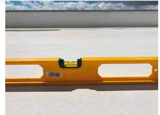
Photo No. 30 – Depicts another view indicating zero slope at the roof structure.
