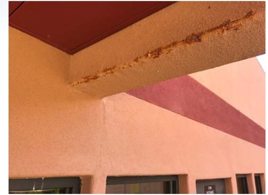
Photo No. 9 – Depicts view at one of several stucco terminations that have prematurely deteriorated due to improper design and installation that has resulted in oxidation of the metal cladding components. A weep screed is necessary at the base of all stucco terminations and transitions and is an important part of a cement plaster stucco wall cladding system.
