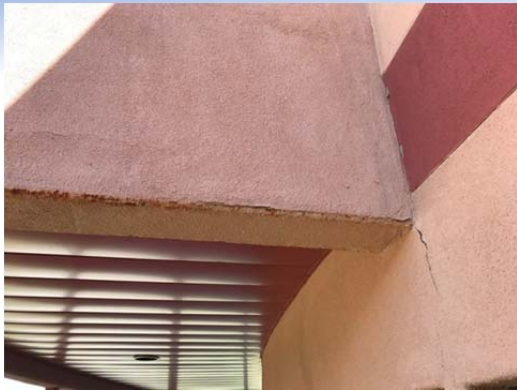
Photo No. 10 – Depicts another exterior stucco transition that does not weep properly, and has suffered severe premature degradation including delamination, cracking, heavy oxidation of metal components, and deconsolidation of the cement plaster.
