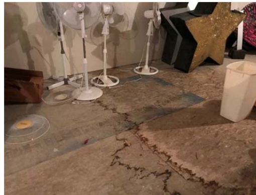
Photo No. 5 – Depicts another detail view at moisture stains in the plywood deck.
