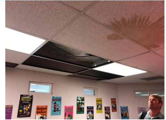
Photo No. 3 – Depicts interior view at the library ceiling that recently experience severe moisture damage from recent snow storms. Staff indicated the ceiling partially collapsed due to moisture related damage.
