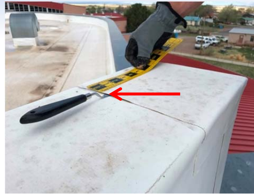
Photo No. 23 – Depicts a fully open flashing membrane seam on a horizontal surface of a parapet. Moisture migration by pressure, capillary action, and freeze-thaw cycles can move large amounts of bulk moisture (i.e., precipitation on the face of the membrane) into the interior of the building.
