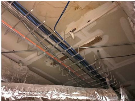
Photo No. 4 – A detail view at one of several moisture stains observed in the unoccupied attic space. Moisture stains were generally observed at or near HVAC duct penetrations through the roof and at roof transitions such as parapet area separate walls.
