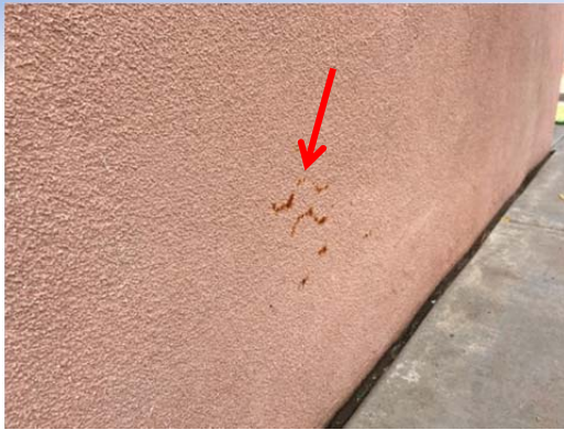
Photo No. 13 – Depicts wire mesh that was not fully embedded in the cement plaster stucco during application. Moisture that migrates through the stucco assembly interacts with oxygen to cause corrosion of the mesh and fasteners that secure this mesh to the wall sheathing. This is an indication of premature failure of the wall cladding assembly and may result in portions of the wall cladding becoming detached from the wall and potentially falling away from the assembly.
