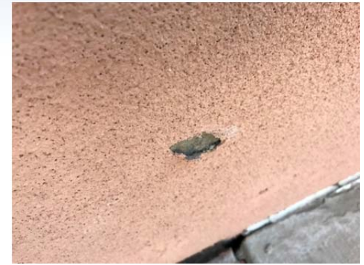
Photo No. 12 – Depicts a detail view at a portion of the wall that has delaminated. This condition is likely a result of poor workmanship during original installation.
