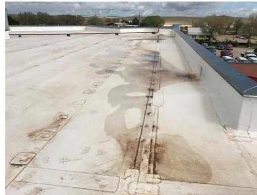
Photo No. 20 – Depicts one of several locations observed this day to have pools of standing water likely a result of zero slope and improperly installed scuppers.
