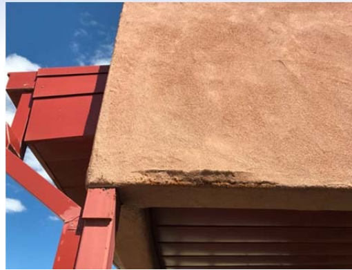
Photo No. 11 – Depicts one of numerous indications that moisture has been trapped within the stucco assembly, cannot properly weep to the exterior quickly as required for this system, and therefore is causing failure of the cladding assembly.
