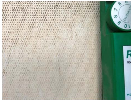
Photo No. 26 – Depicts detail view at one of several locations in the field of the membrane observed to have micro-splits. This formulation of TPO membrane was flawed during manufacturing and the result is splits that allow moisture migration through the membrane.
