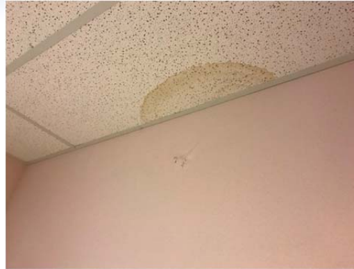
Photo No. 2 – Depicts one of several moisture related stains at the building interior, observed during an initial interior walk-through guided by facility maintenance staff.
