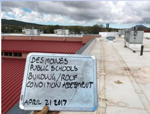
Photo No. 16 – Depicts overall at a portion of the single ply TPO roof surveyed this day.
