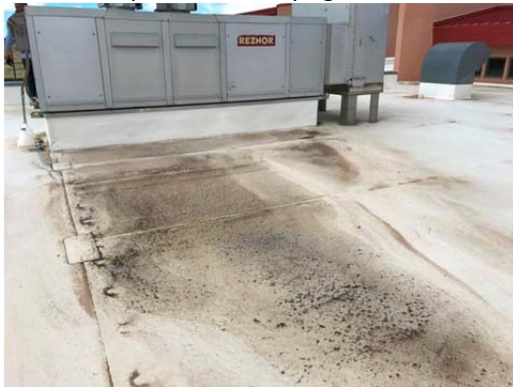
Photo No. 34 – Depicts the HVAC unit above the library ceiling that has recently collapsed due to moisture intrusion. Membrane flashing at the support assembly is not properly terminated, and micro-splits as well as improperly welded seams in and adjacent to ponding water is likely the source of moisture intrusion.
