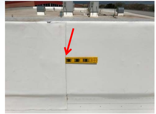
Photo No. 24 – Depicts a large vertical parapet flashing membrane seam that is open. The membrane material does not appear to have been fully heated to get a proper welded seam. This condition is likely a result of poor workmanship during installation.
