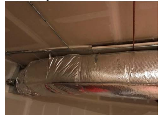
Photo No. 6 – Detail view at a duct penetration through the roof that was observed to have damaged the ceilings thermal barrier board sufficient to partially collapse. This condition has compromised the building fire protected assembly and should be repaired as soon as possible.
