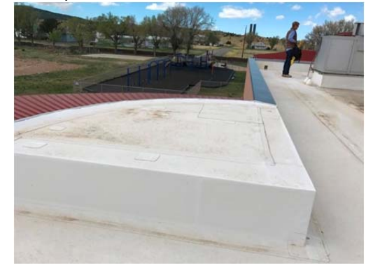
Photo No. 36 – Depicts a portion of the building transition that is covered with roof membrane as waterproofing. This and other irregularities in the building add complexity to a reroofing design.
