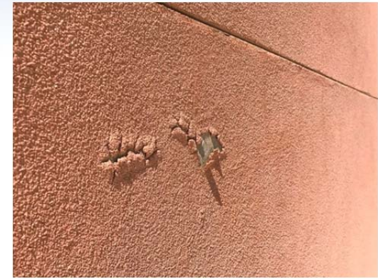
Photo No. 15 – Depicts one of several moisture blisters that have resulted from trapped moisture at a stucco cladding assembly that has been coated with a non-breathable, vapor impermeable coating. Stucco cladding systems by design permit moisture migration through the cement portion of the system, that must then be redirected to the exterior using rigid flashing, weep screed, and a properly formed watertight WRB membrane.
