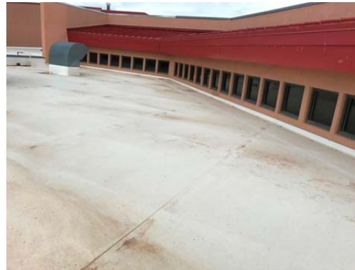
Photo No. 35 – Depicts clerestory windows that are installed adjacent to the roof system, with insufficient clearance to properly terminate the membrane minimum 8-inches above the membrane. These windows are problematic for new tapered insulation that is required to properly slope the roof if a low-slope roof system is selected for replacement.
