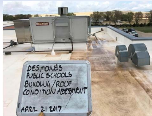
Photo No. 17 – Depicts a typical curb mounted HVAC assembly adjacent to large areas of roof material observed to have sediment and ponding water, indicating long term standing water is present at the roof frequently.
