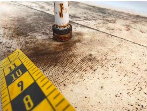
Photo No. 25 – Depicts one of several roof penetrations that does not have a properly formed flashing boot, membrane seal, and termination that must be minimum 8-inches above the field membrane.
