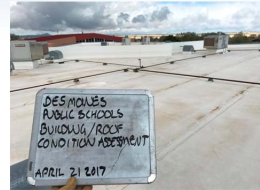
Photo No. 18 – Depicts overview at a large field area of single ply TPO roof membrane. The membrane is mechanically fastened to the roof deck, as indicated by sediment stains that have accumulated around indentations made by the fastener plates at each seam.
