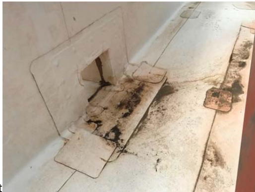
Photo No. 19 – Depicts one of numerous through wall drainage scuppers observed to have large pools of standing water adjacent to the opening. This is likely a result of poor workmanship during initial installation.
