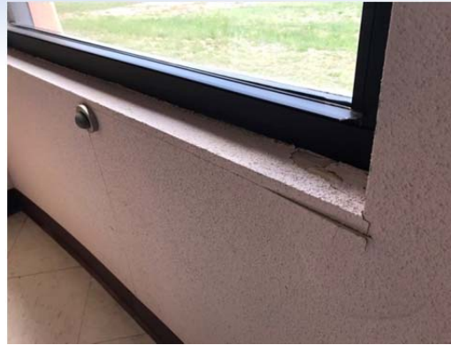
Photo No. 8 – Depicts detail view at one of numerous aluminum framed storefront window assemblies observed to have moisture related damage. This condition can result from interior condensation on the cold frame, and may be a result of poor workmanship at the window rough opening flashing and exterior seals during original installation.
