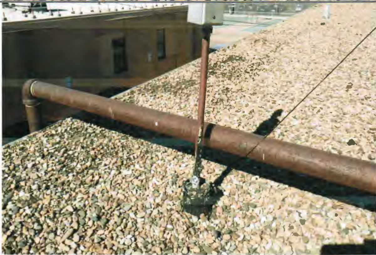
ACM Roof penetration tar.
