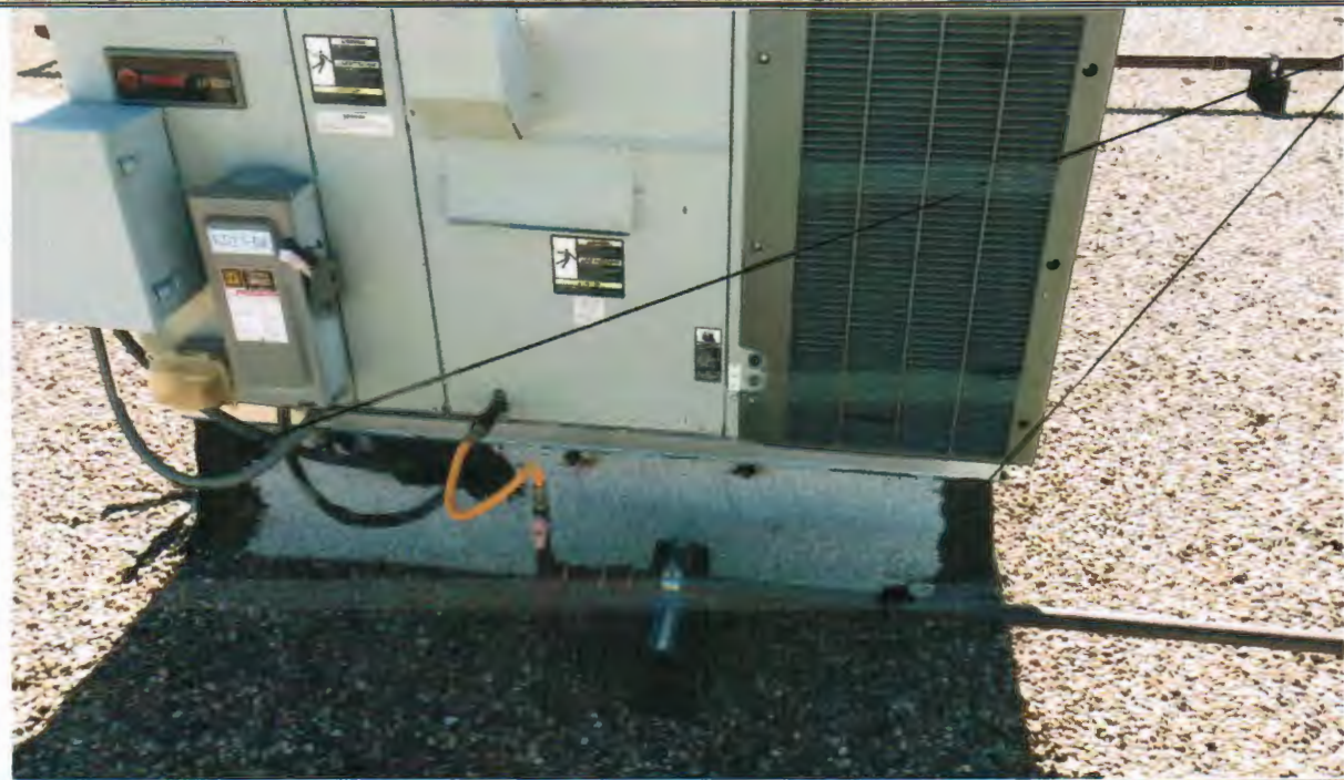
ACM Rolled roof seam tar on HVAC flashing.
