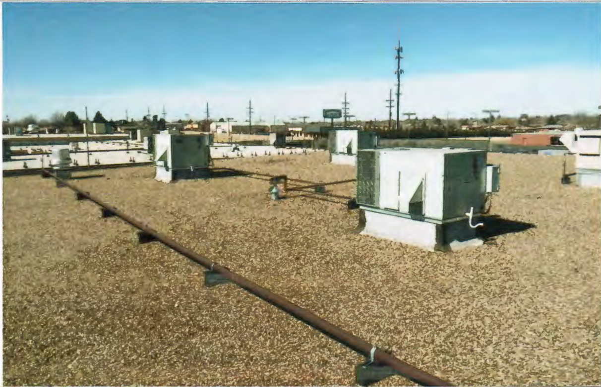
G-Wing, Upper Tar and Gravel Roof.
