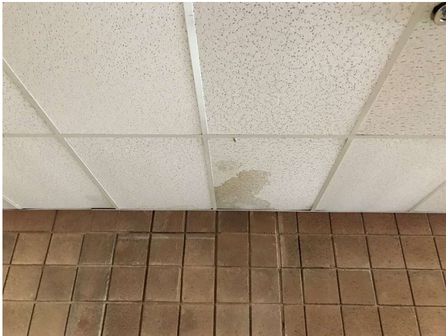
Figure 2 - Example of leak investigation
