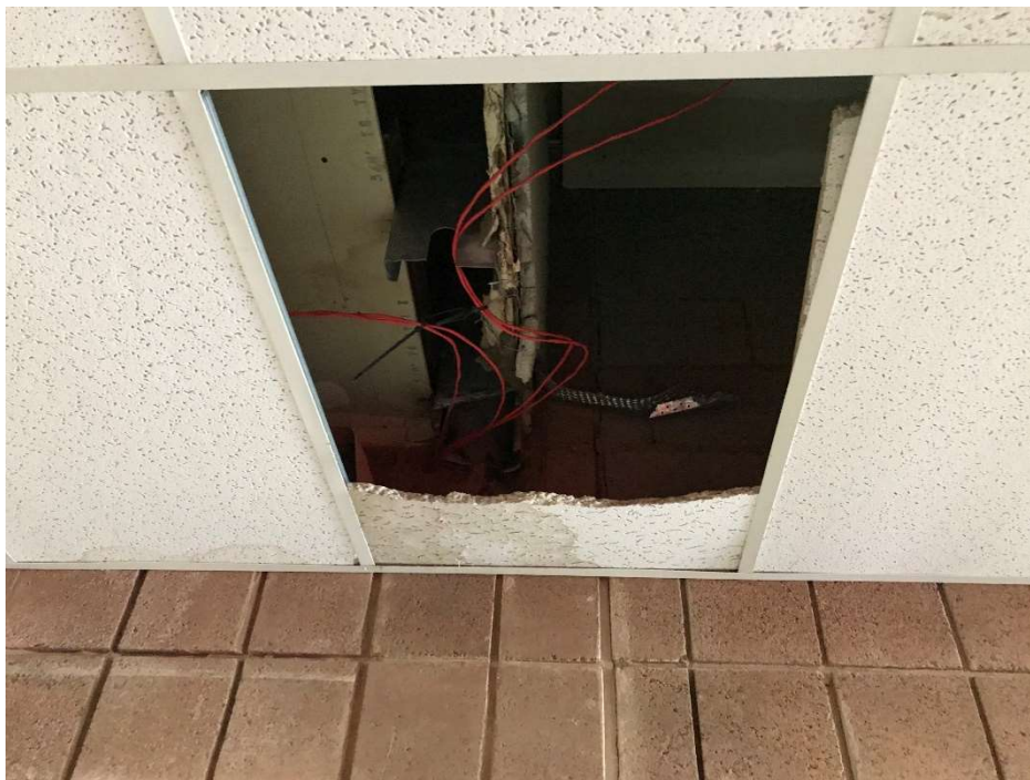
Figure 3 - Internal damage from leak
