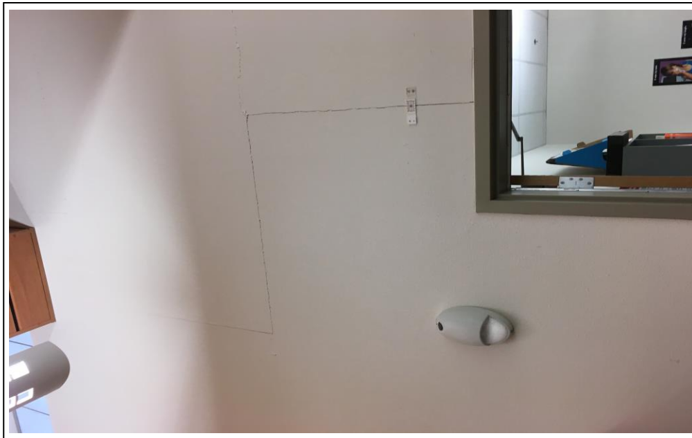
Photo 6: Wall Crack with Crack Gauge
