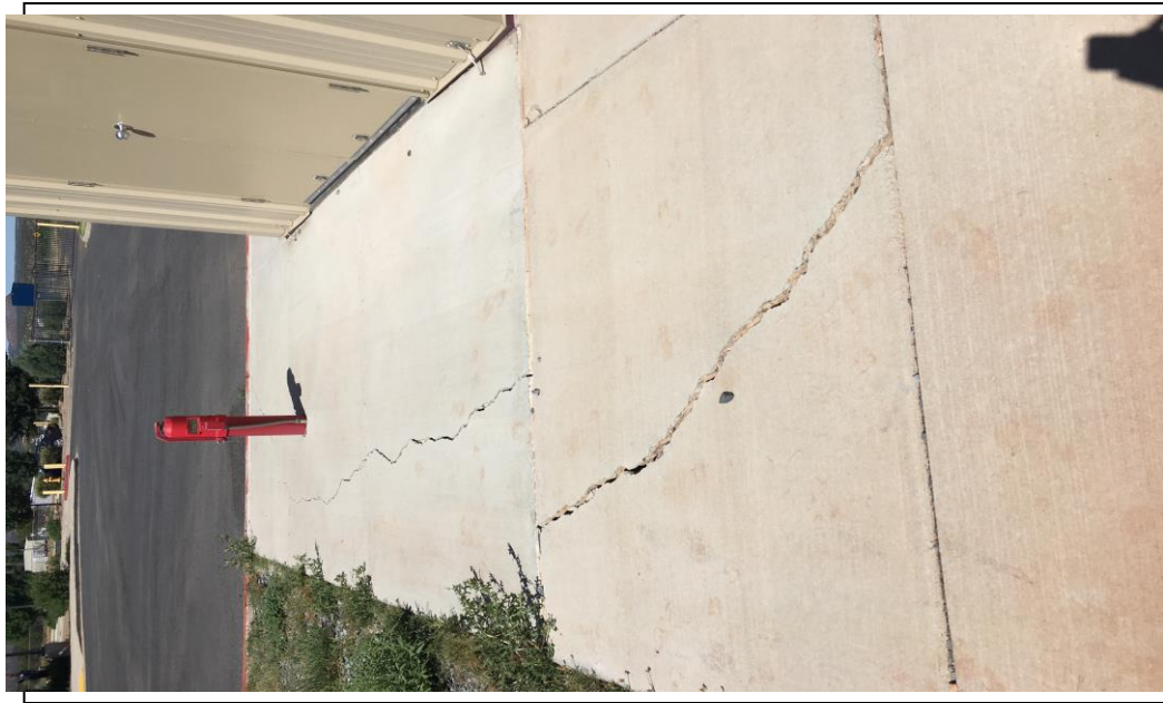
Photo 11: Site Flatwork Cracking
