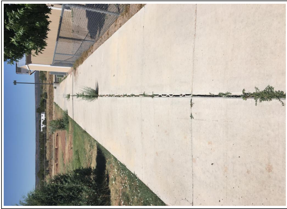
Photo 13: Site Flatwork Cracking/Separation
