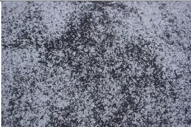
Severe Granule loss to surfacing membrane
