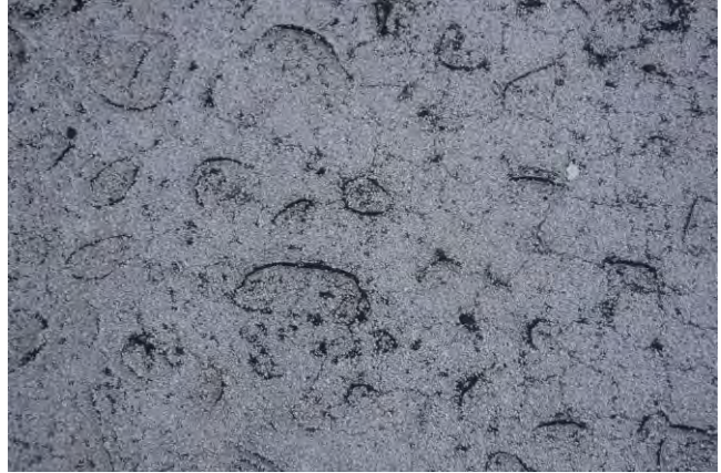
Closeup of blistering at seams and laps
