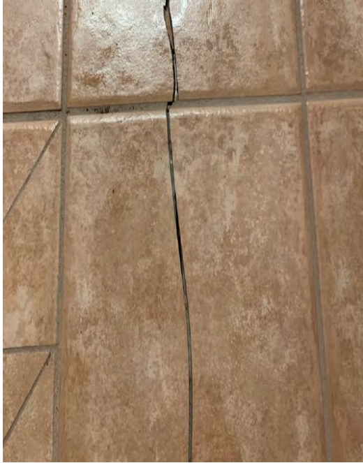
Picture of floor shifting in 2002 building.
