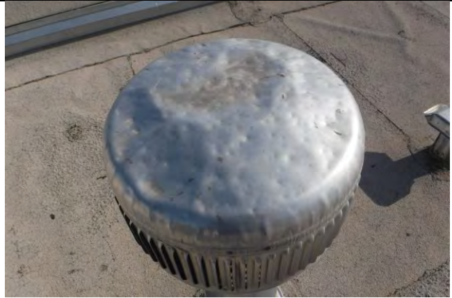
Evidence of possible hail impact damage to soft aluminum vent caps
