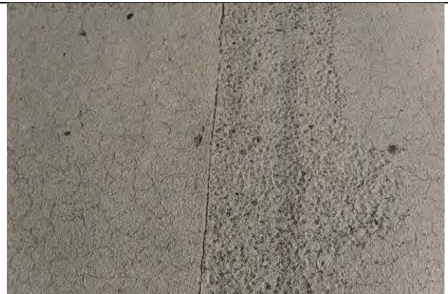
Small blisters /bubbles at seams and laps
