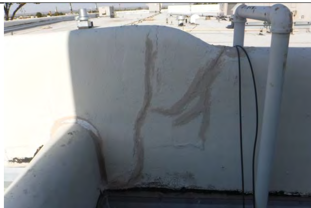
Cracks in Stucco wall
