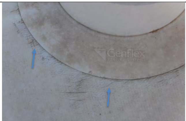
Small splits in membrane near penetration boots
