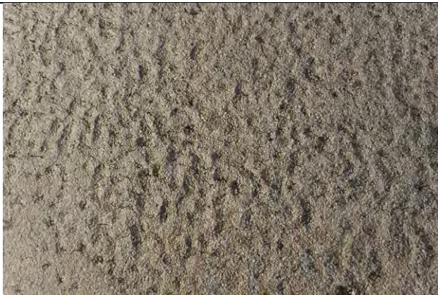
Close up of small blisters/bubbles at seams and laps causing separation and granule loss
