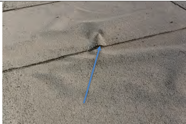
Blister at seams creating a leak entry point
