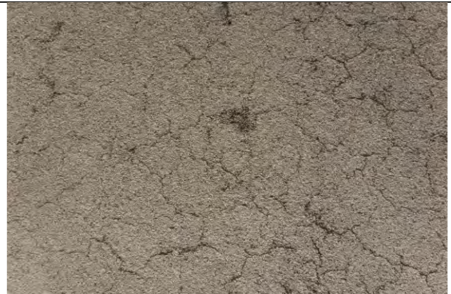
Surface Membrane alligatoring
