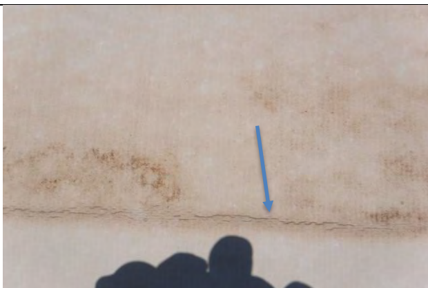
Splits in TPO at insulation joints
