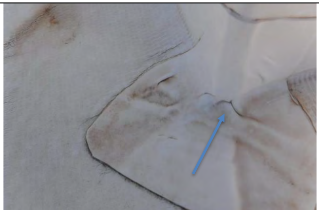
Splits in TPO at corner detail
