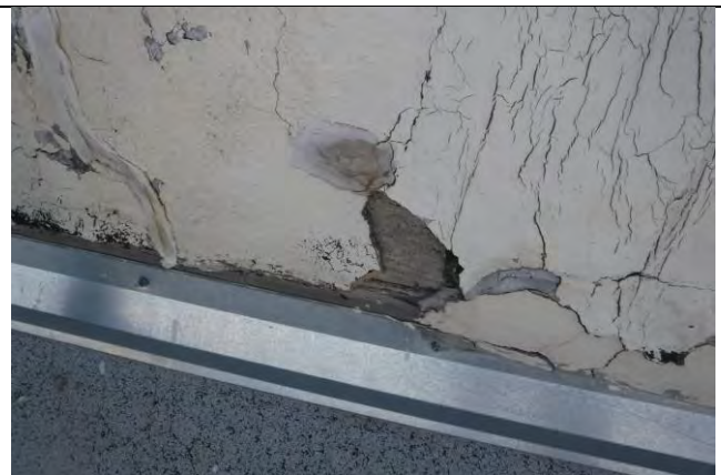
Deteriorated stucco at parapet wall
