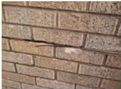
Rusted Horizontal Reinforcement
