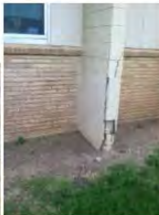
Cracked CMU Wing Wall
