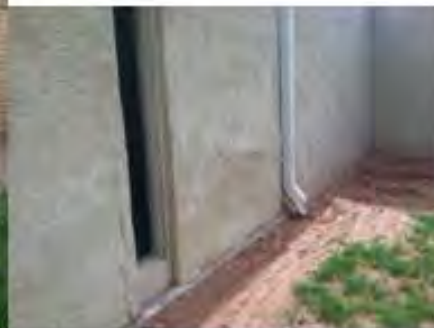
Stucco Deterioration
