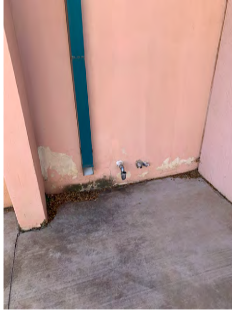
Damaged Plaster
