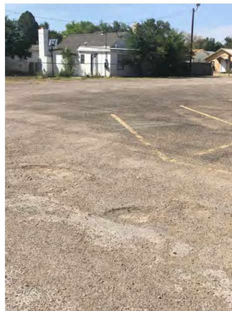
Exposed Subgrade in Existing Parking
