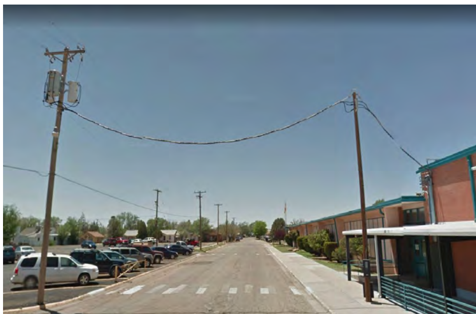
Brown ECC Existing Primary Power Pole, Secondary Power Pole
