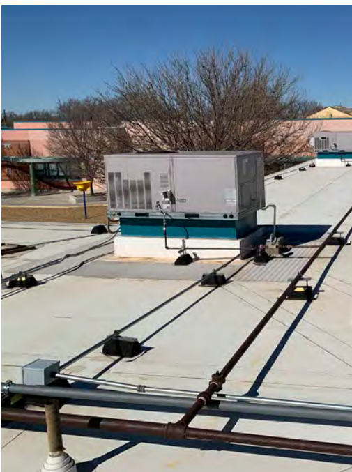
Typical Existing Roof Top Unit
