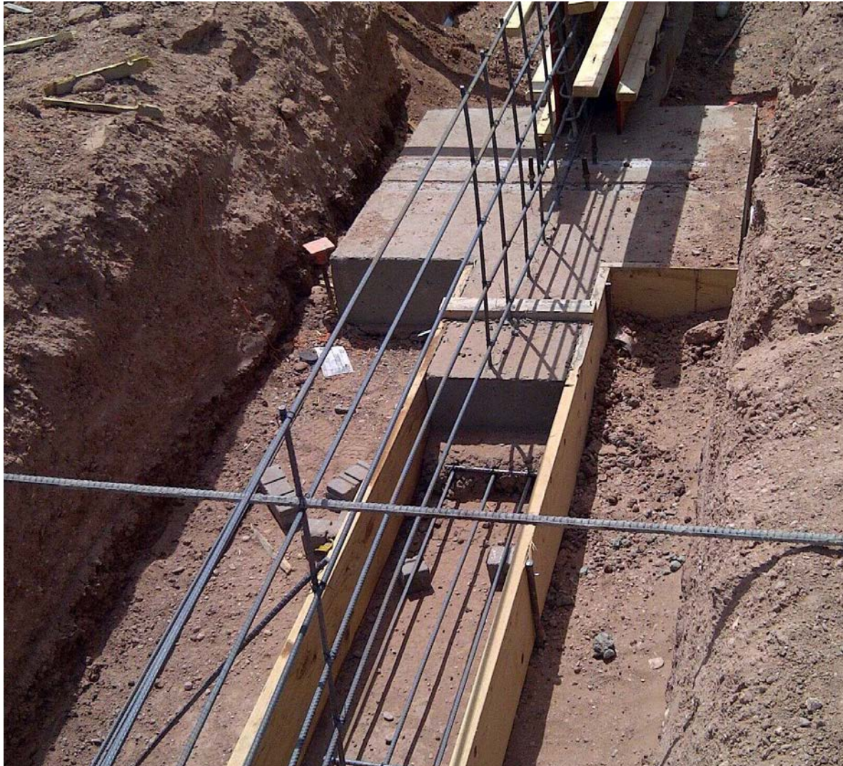
Photo 5 Bottom of Footing Conditions 04/16/2013
