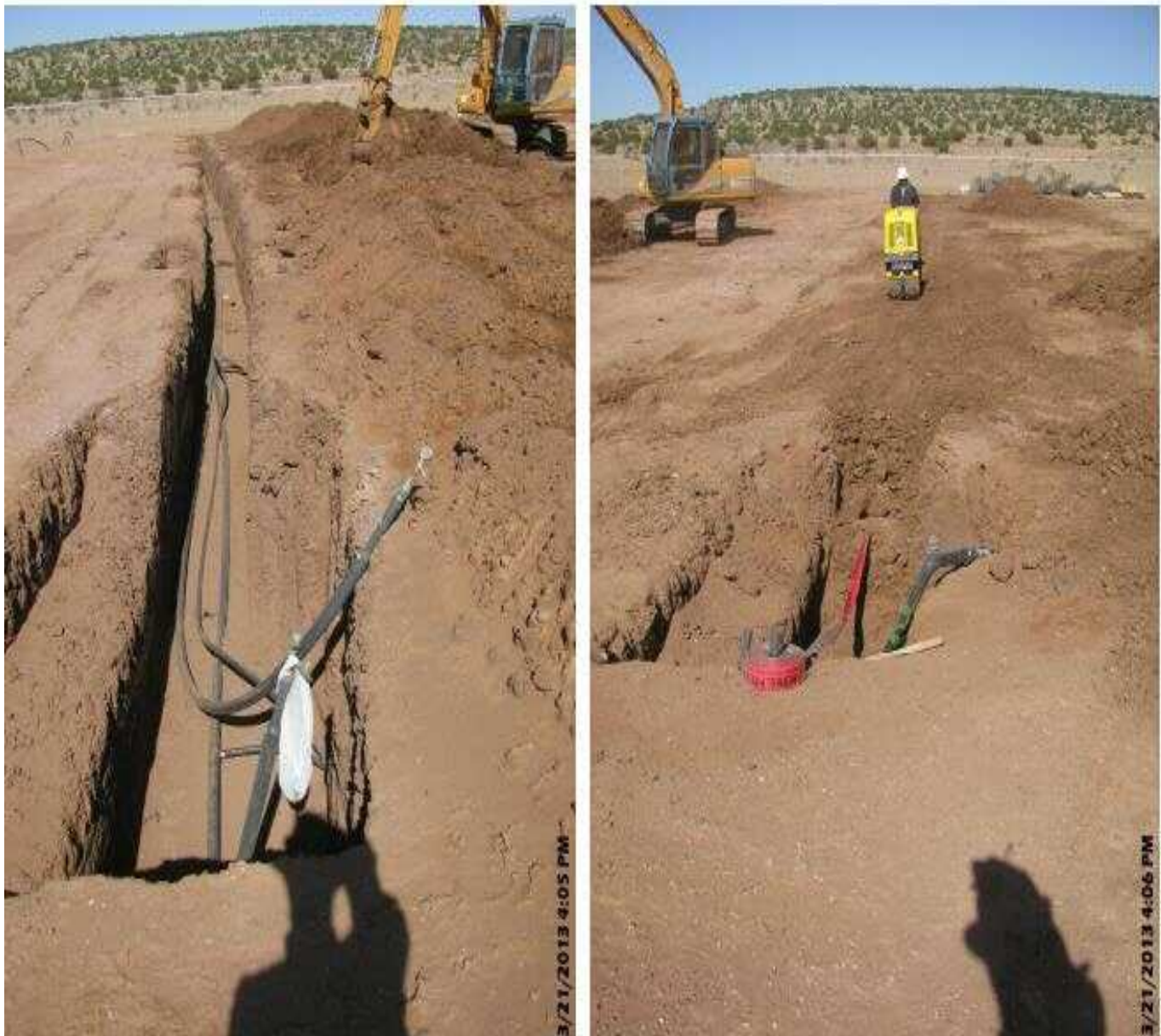
Photo 4 Excavation/Backfill in Native Soil-Geothermal Piping
