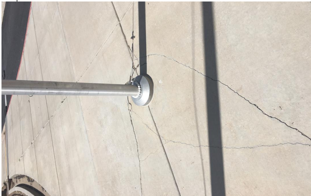
Photo 8: Site Flatwork Cracking
