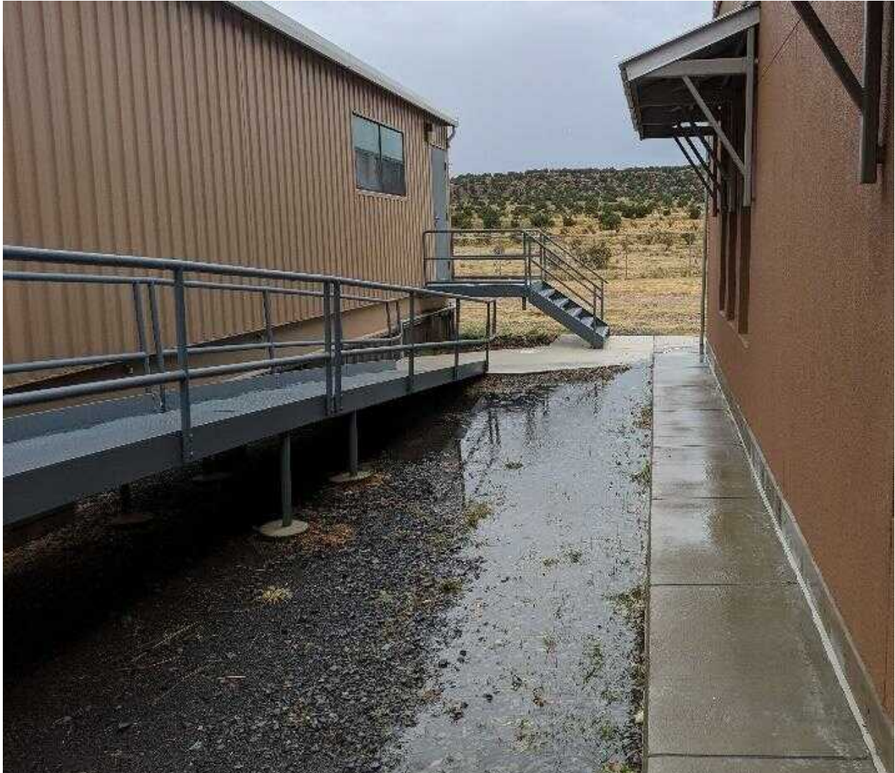
Photo 6 North side of building ponding water
