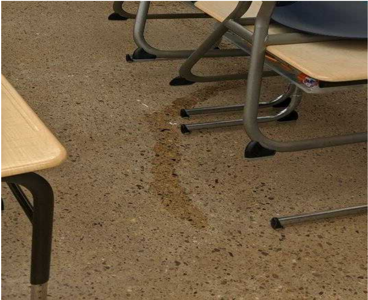
Photo 7 Water Streaming into Learning Lab Room 133
