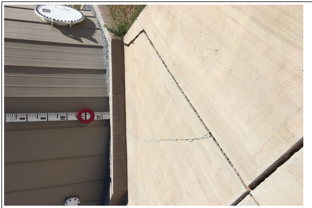
Photo 10: Site Flatwork Cracking
