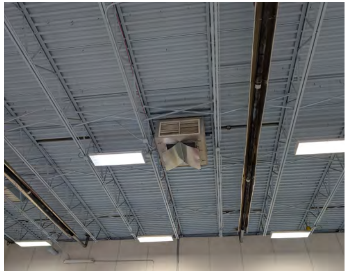
Below: Gymnasium Gas Fired IR Heaters and Evaporative Cooler Distribution
