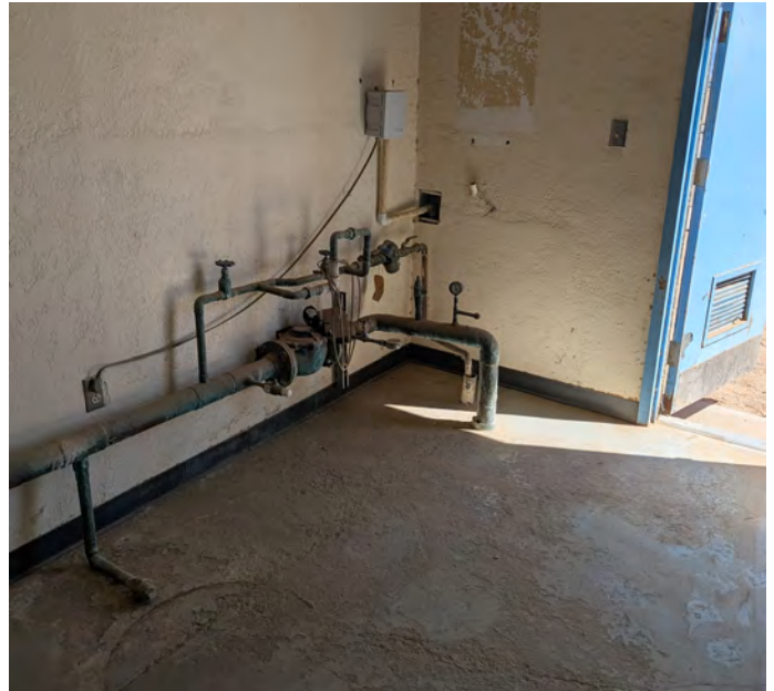
Above: Domestic Water Entrance Below: Typical Domestic Hot Water Heater
