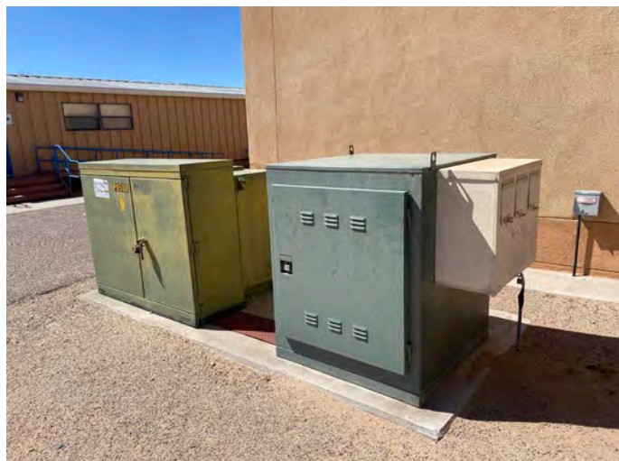
Above: Main Electrical Room Below: PNM Service Transformer and CT Cabinet
