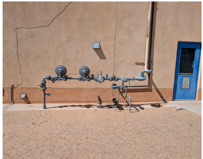
Above: Typical primary and secondary roof drain system Below: Natural gas meter and regulator assembly
